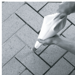
Figure 22 - Grouting Brick
